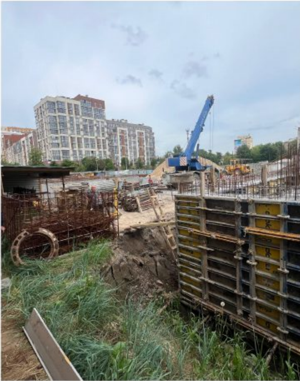
Foundation formwork
