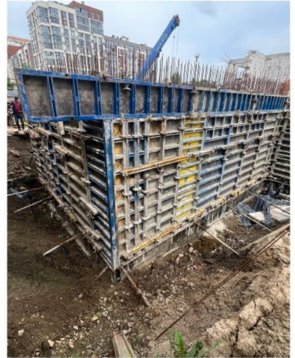
Concrete structure in progress
