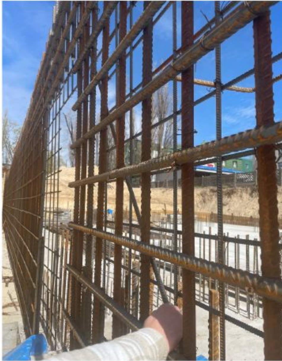
Wall reinforcement
